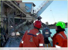
Surveyors preparing the 3D laser scanning of the deep-excavator
